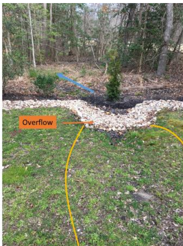
Before: Overflow location and flow Path (blue arrow)
