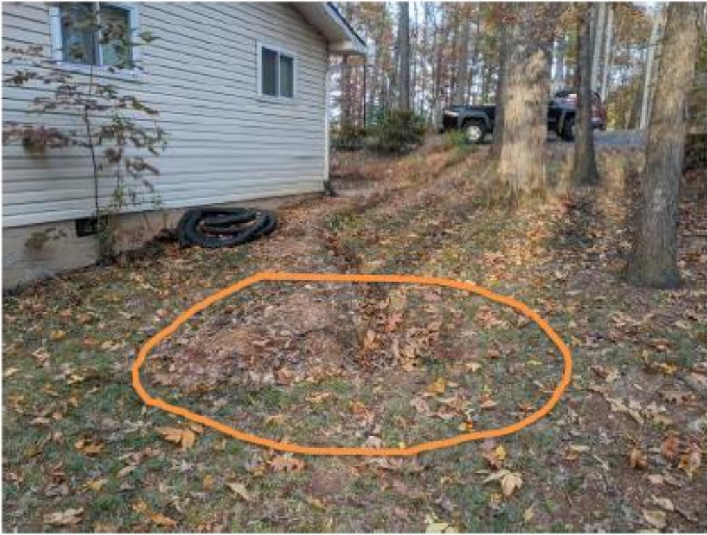
Side yard view of possible Dry Well location. Also shown is the poorly done work by previous contractor.
