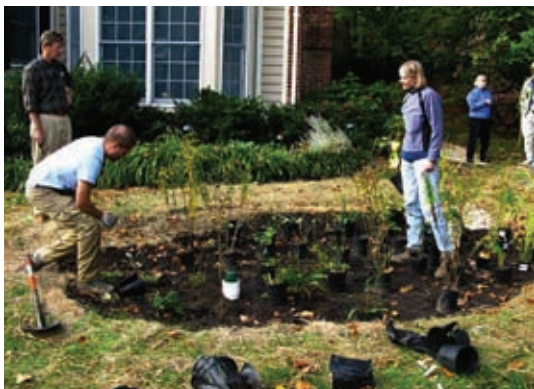
Native plants are placed in a rain garden in Falls Church.
